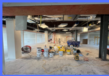
2nd floor with new concrete deck
