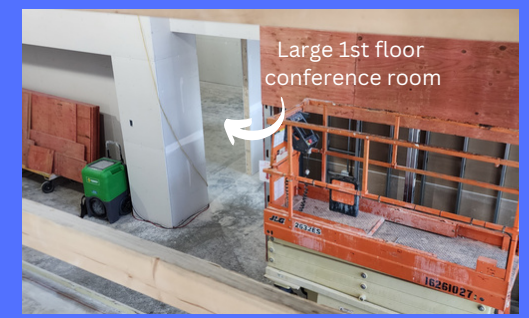
1st floor view from the Mezzanine
