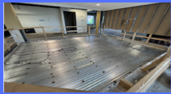
2nd floor decking for expansion
