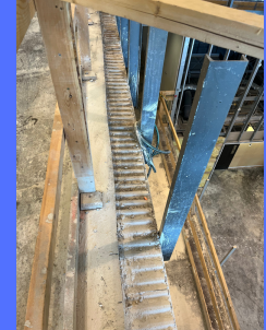
Prep for 2nd floor concrete deck
